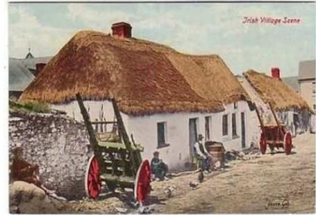
For over 9,000 years, thatch has been used as a roofing material in Ireland especially on Irish Cottages. Nowadays, the difficulty of finding people to do the thatching, the further difficulty of acquiring insurance for thatched Irish cottages, the need for continual maintenance of this roofing material, and the availability of cheaper more durable roofing have all mitigated against the preservation of this important part of our heritage.
